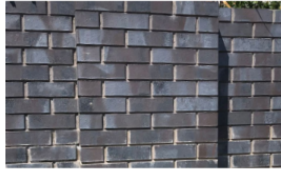
Brick type 1 Dark Grey Brick (CLA101) Handset, conventional brick recess Mortar ref: 021
