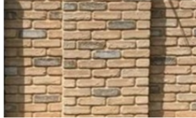
Brick type 2 Light Buff Brick (CLA102) Handset, conventional brick recess Mortar ref: M3WLK34
